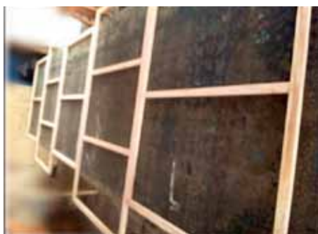
Figure 9. The constructed wooden frames. Source: Studio Work (2021).
